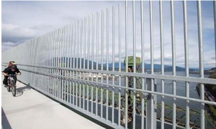
Figure 6.12 Iron Workers Memorial Bridge, Vancouver
