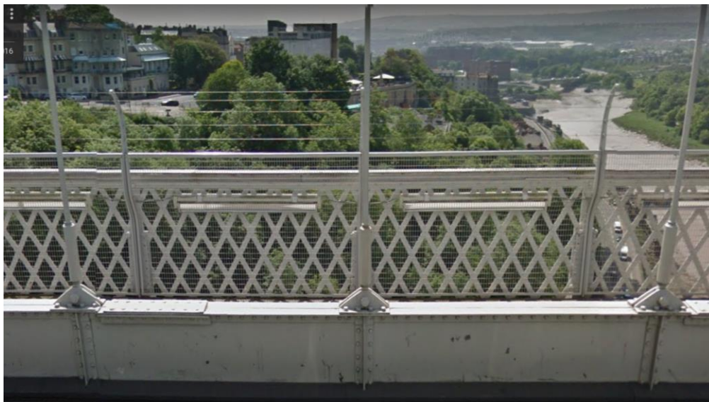
Figure 5.3 Elevation of the parapet and the minimal visual impact from this view
