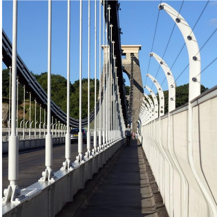
Figure 5.2 View along the footway showing the inclined barrier
