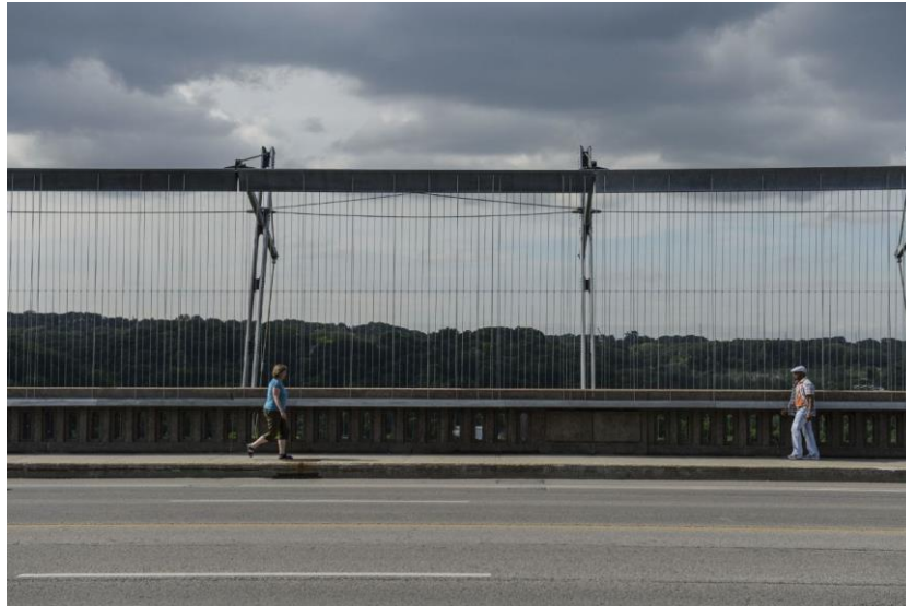
Fig 5.1 Bloor Street Viaduct Barriers
